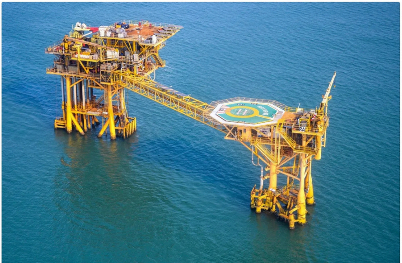
An offshore platform at Cairn's Ravva asset. (Photo: Cairn Oil & Gas)
